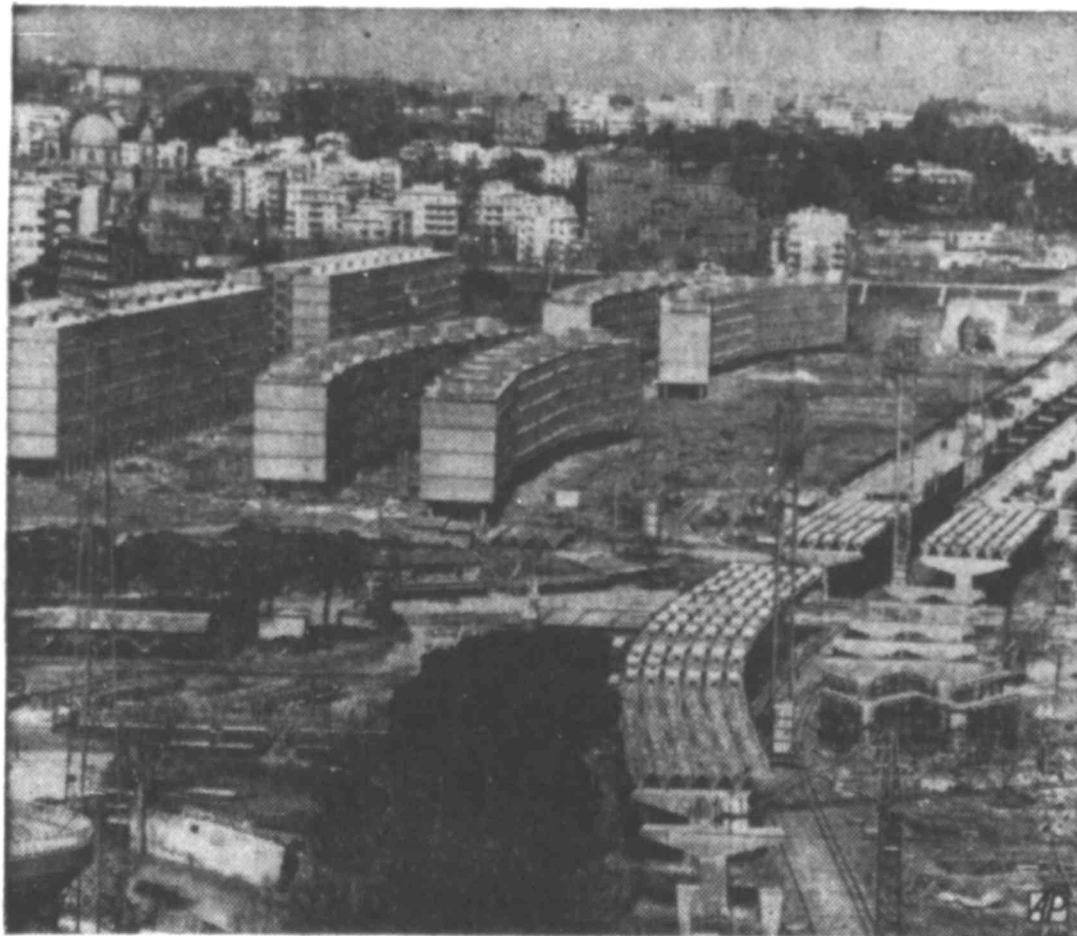
OLYMPIC VILLAGE AREA — The construction of the Olympic Village at Rome is in the final stages. Elevated highway at right is being built to link all phases of the Games. The blocks of apartments at left will house competitors from all nations.
