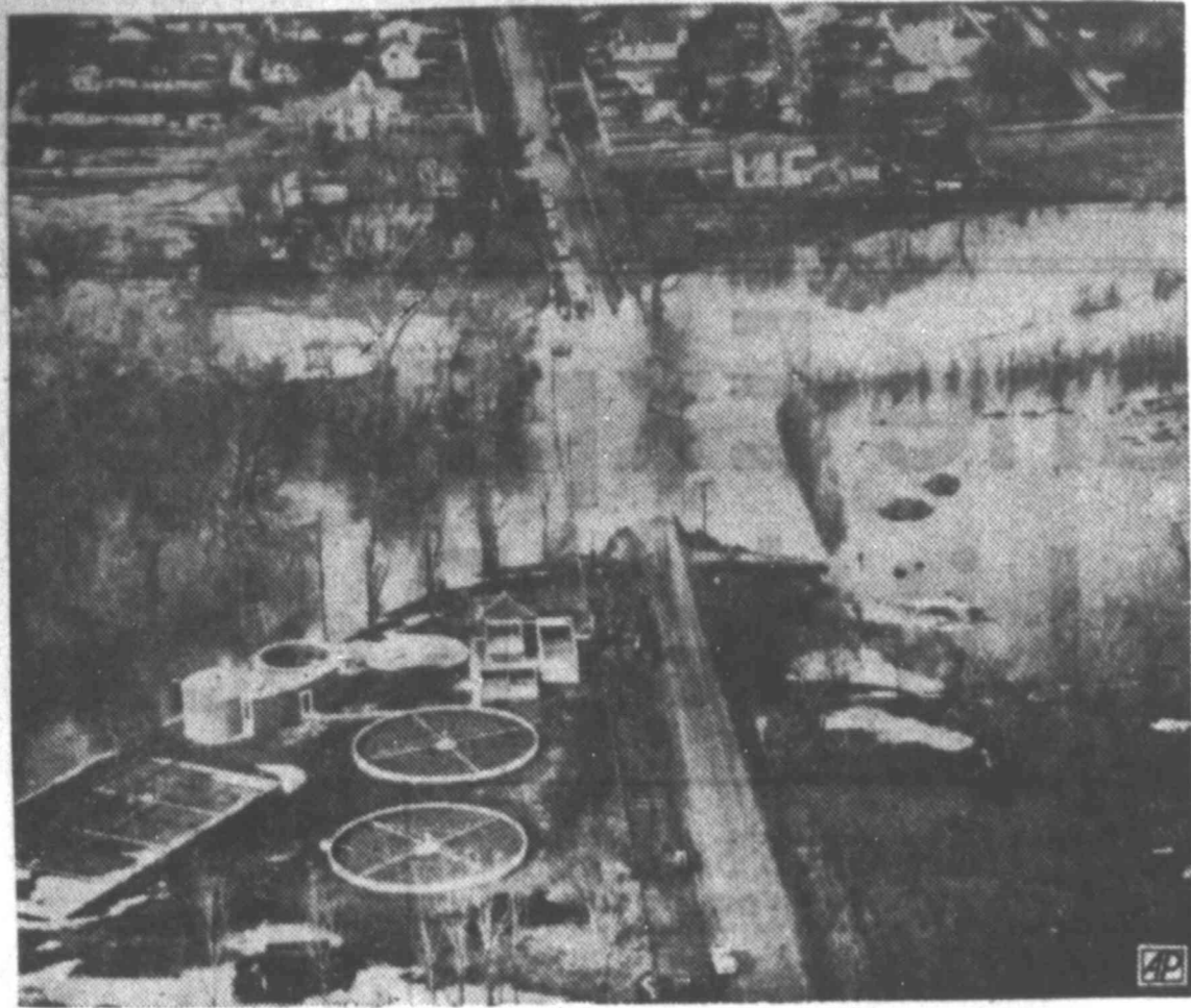
Flood Waters Block Highway
