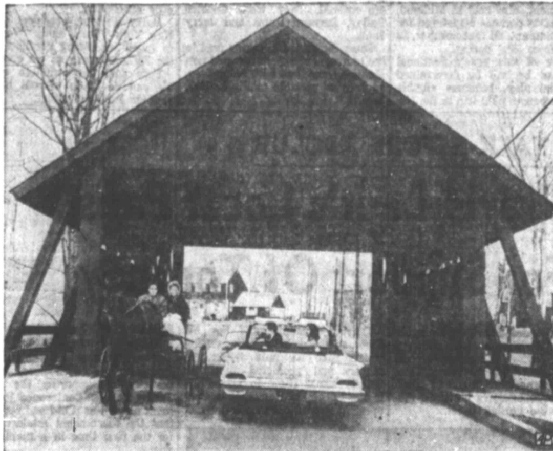
THE PAST RENEWED — A meeting of two eras is symbolized by the horse and buggy and auto at the covered bridge over the Cooper River in Delaware Township, N. J. However, this bridge, reminiscent of the past, is different. It was just built.
