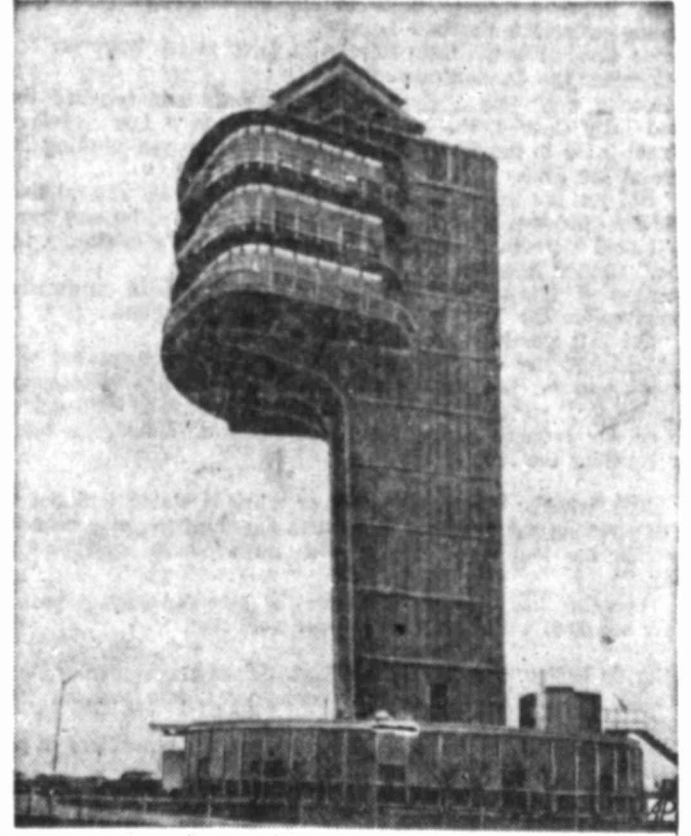
TRAFFIC CENTER — This is the new 150-foot concrete control tower where a crew of 89 men direct the flights in and out of the busy Newark, N. J., Airport.
