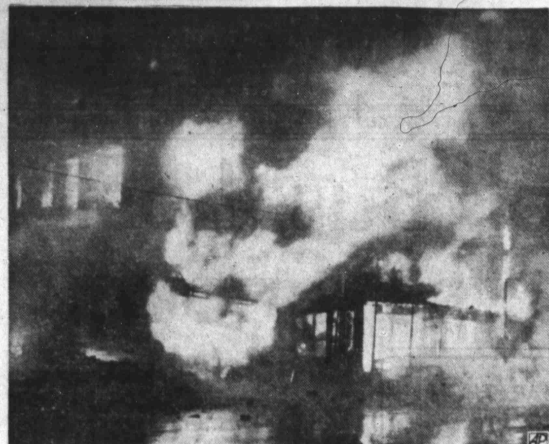
Fire Destroys Downtown Buildings
