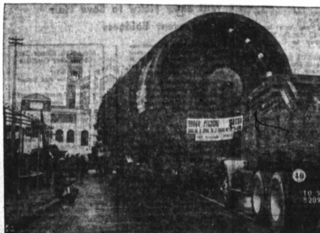
REAL SLOW FREIGHT —A 240-ton boiler is transported around bend of street in Nettuno on its way to Italy's new nuclear plant at Laina. The special truck trailer, hauling the boiler, moved at an average speed of less than a mile an hour.
