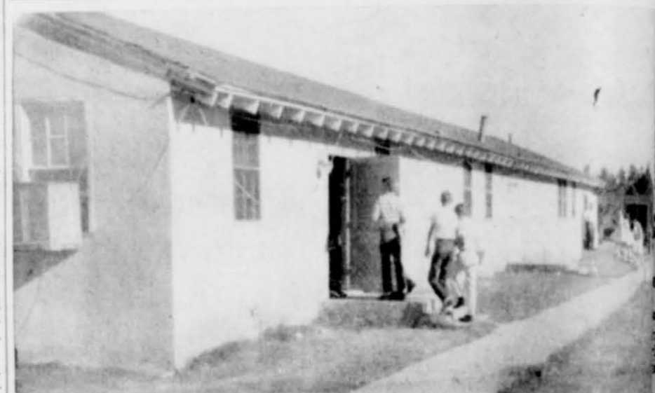
BAND HALL—This is the band hall at Dimmitt High School, a converted Westinghouse building. It is totally inadequate in size, lighting, acoustics and other considerations. School officials who have arranged for a new, modern band hall in the present school building to be decided on in a bond election October 7.
