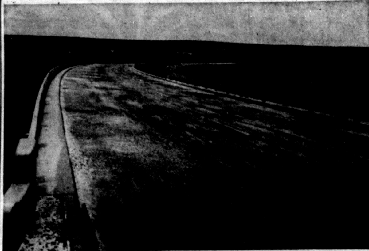
FM 700 LOOP COMPLETED AS AN AID TO HEAVY TRAFFIC Connection between US 80 and US 87 was completed and put in service
