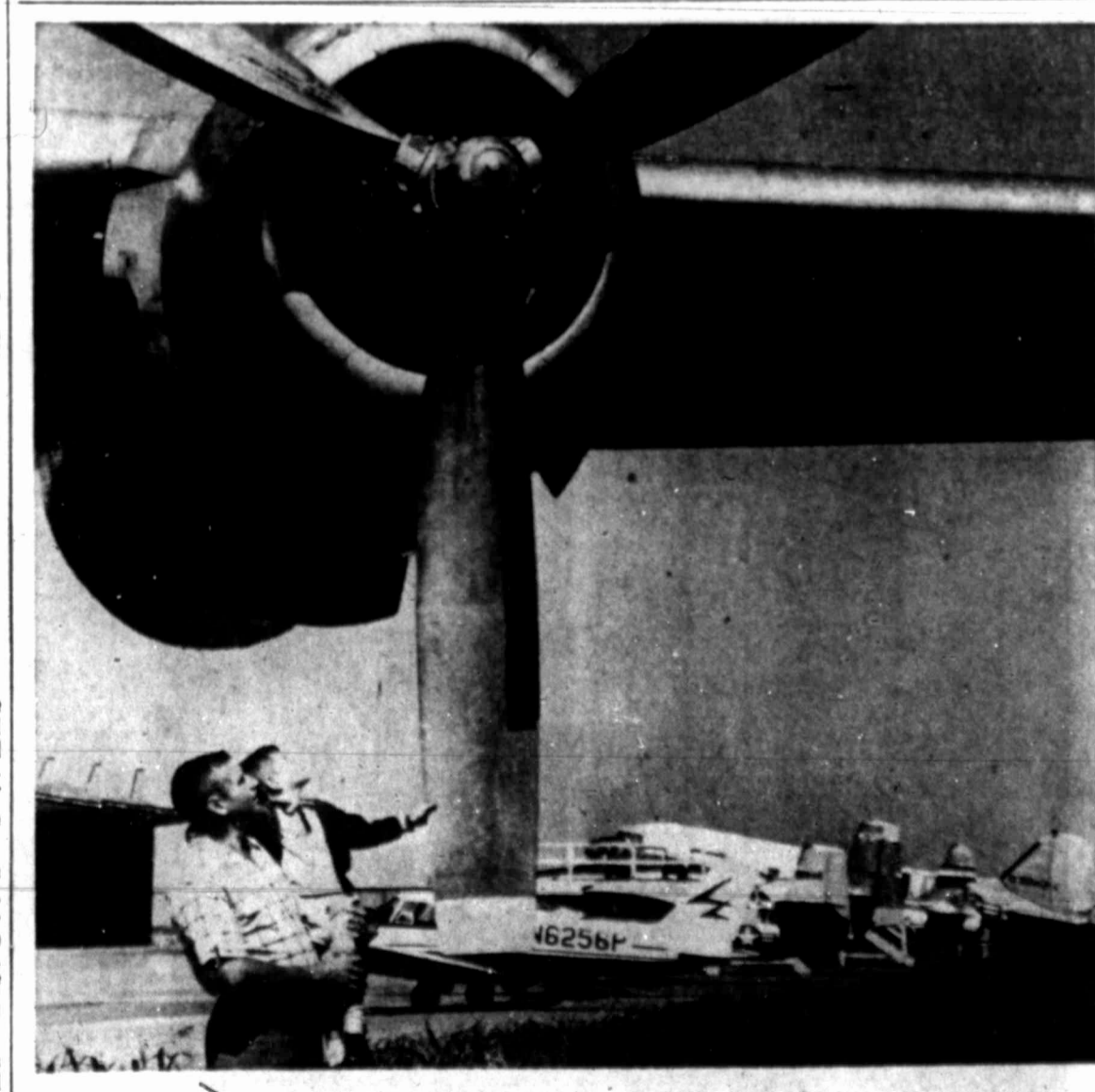
New Airport Is Dedicated
