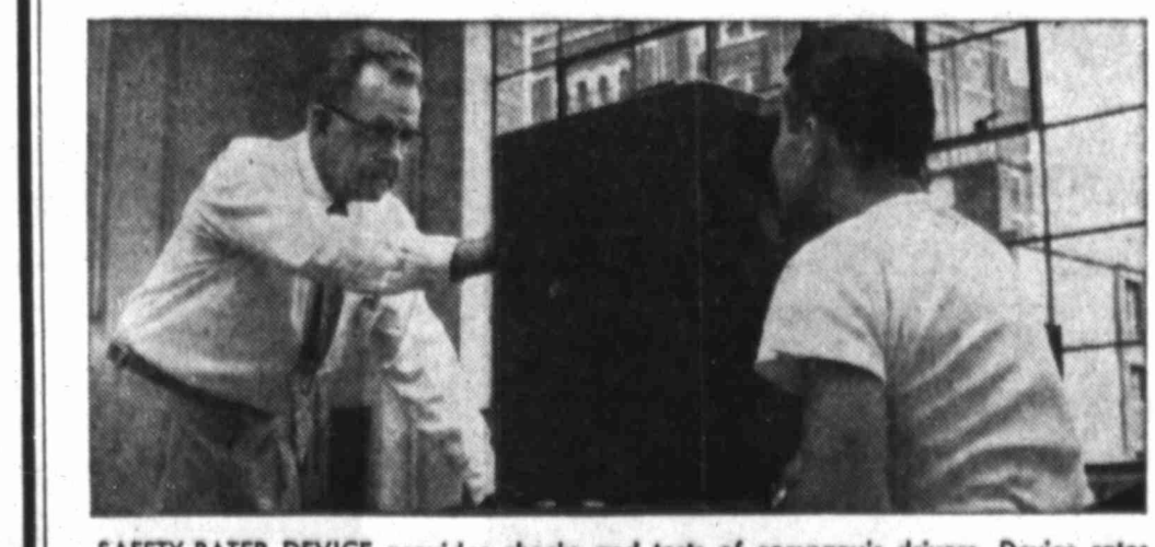
SAFETY-RATER DEVICE provides checks and tests of company's drivers. Device rates reflexes and vision, points out weaknesses that practice and extra caution can overcome.
