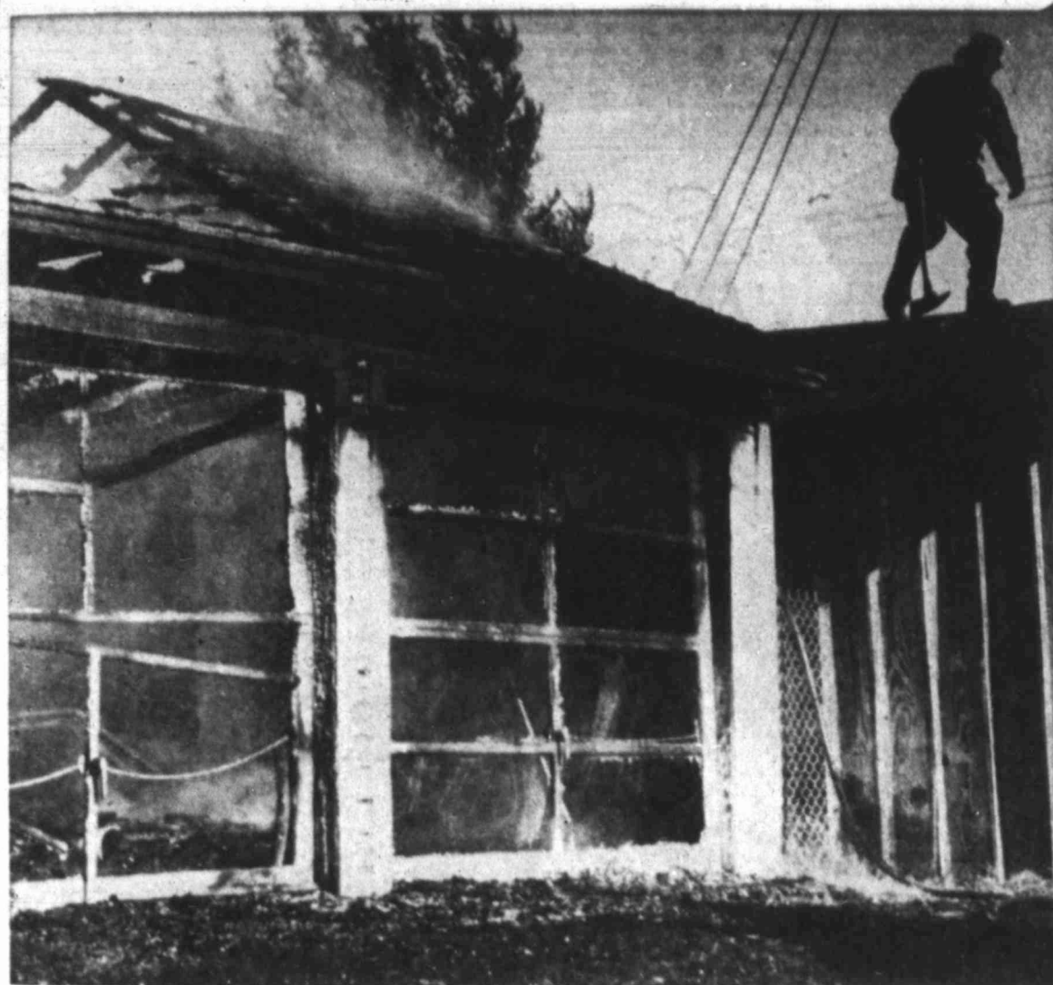
Garage Levelled By Blaze
