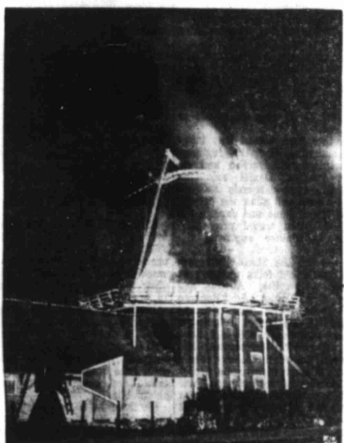
TRICK SIGHT — The light bulbs installed on vanes of this old Dutch mill near Amsterdam and the cameraman's time exposure create illusion of high speed.
