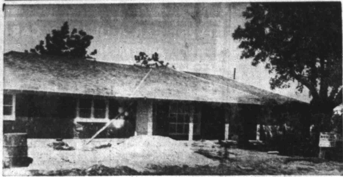
TYPICAL STANTON CONSTRUCTION ... Fine Homes, Modern Business Buildings
