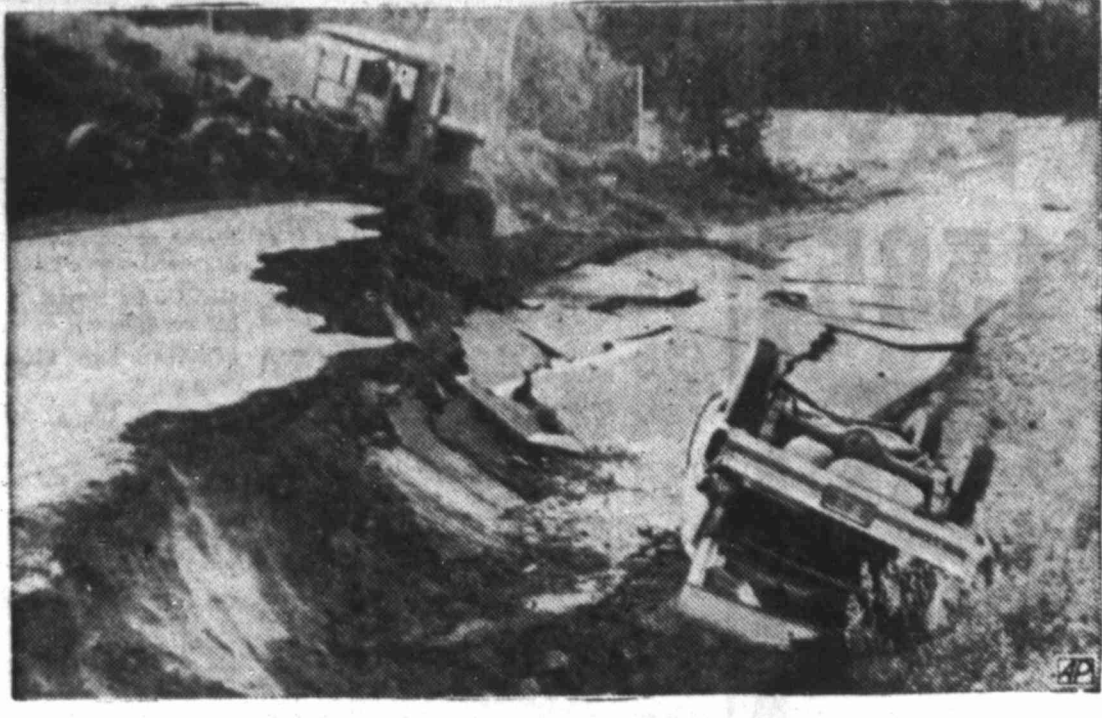
Earthquake Rips Highway
