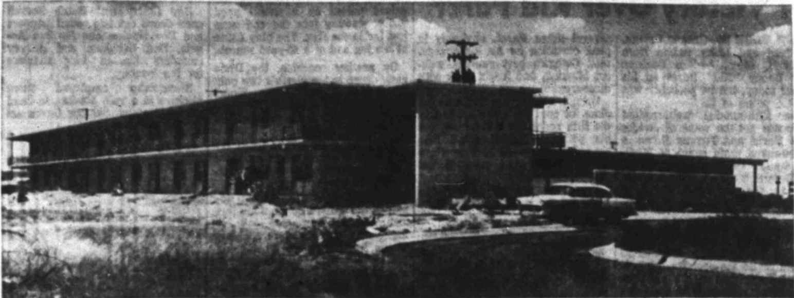
HCJC's New Dormitories To Be Ready For Occupancy Finishing touches to the two new dormitories at Howard County Junior College are under way. All ready applications are being received for rooms in the dormitories. College officials urge that any student who wants accommodations file his request at once. The dormitories are modern in all details and remarkable for their attractiveness and the conveniences which are incorporated in them for the comfort of the students.
