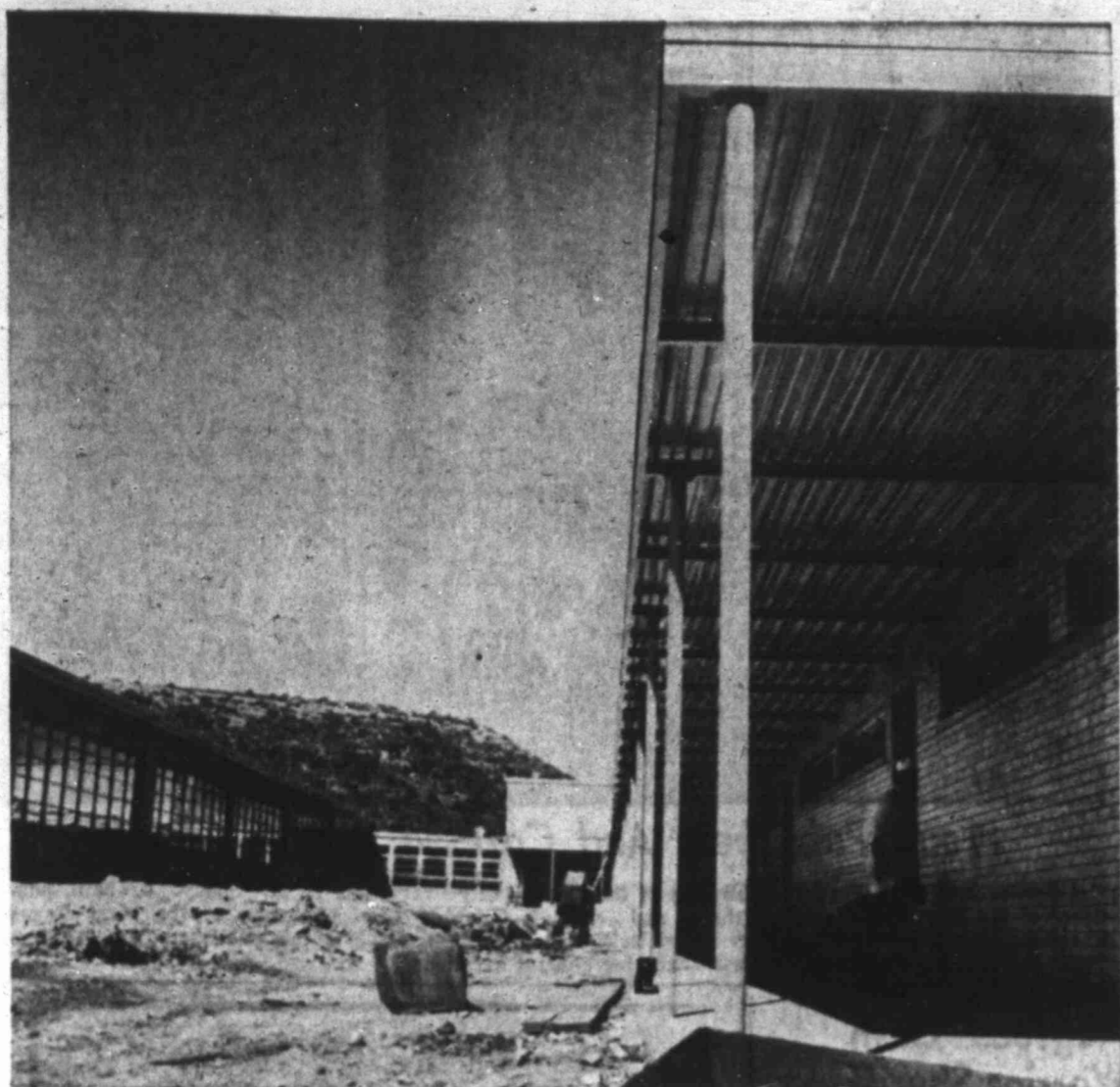
More Classrooms For Park Hill School
