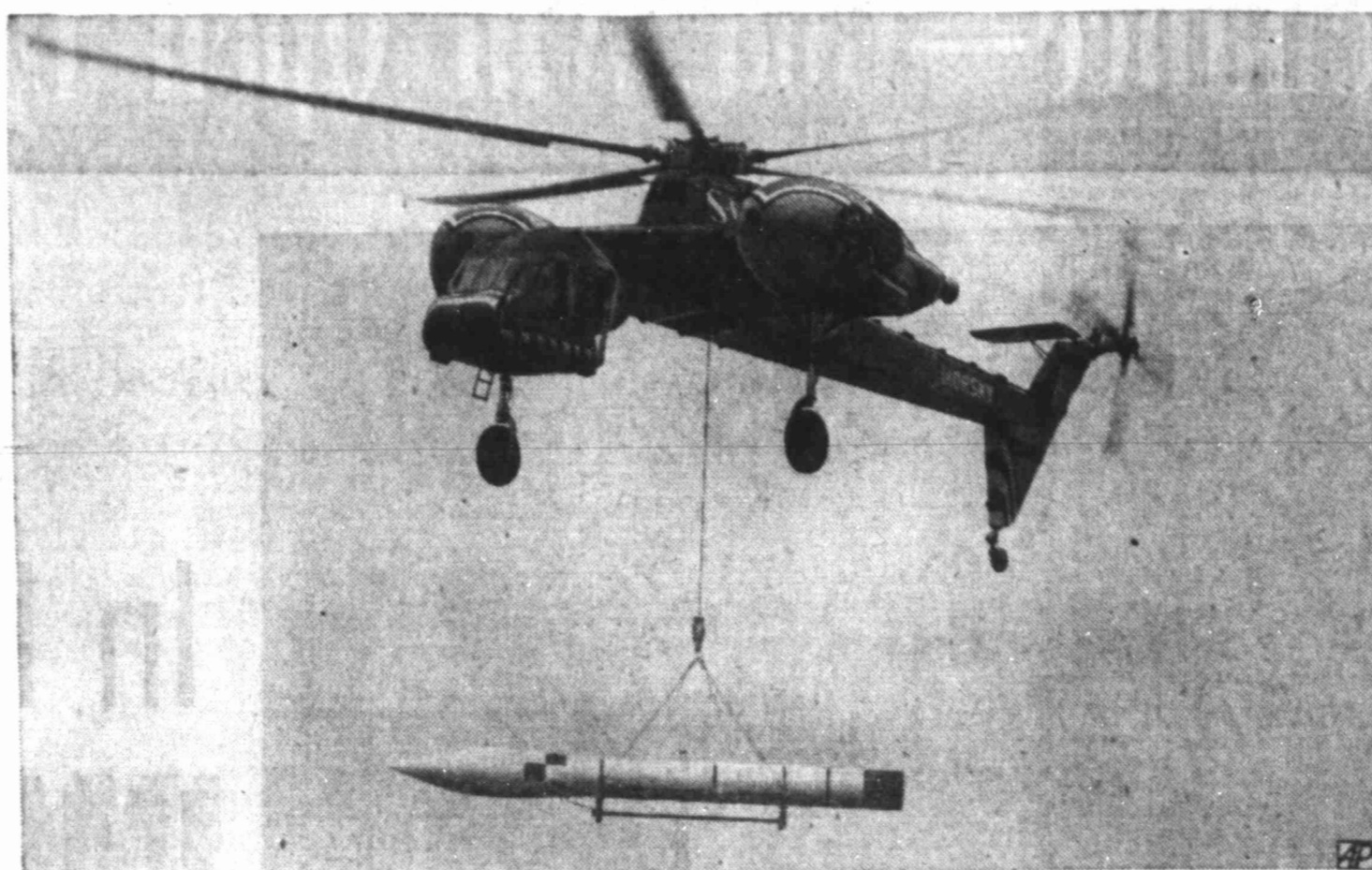
LOOKS AREN'T EVERYTHING —Helicopter, minus usual fuselage but with five-bladed rotor, totes dummy rocket at Stratford, Conn., in first public show. Sikorsky-built 'chopper can tote six tons, making it a real skyhook.
