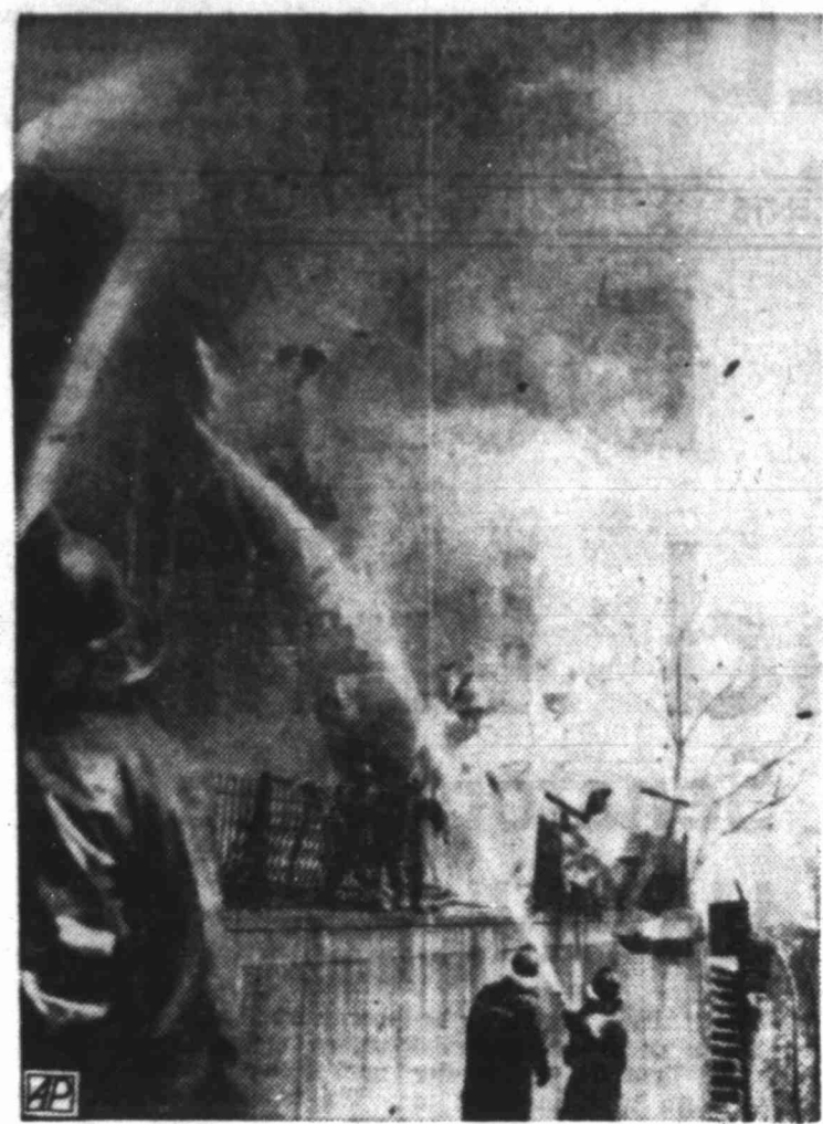
Debris Rains On Firemen
