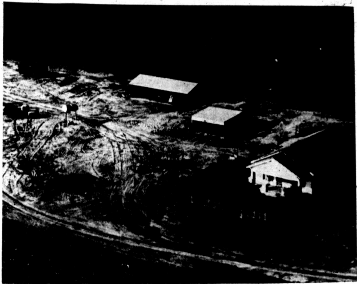
FARM HOME OF MR. AND MRS. E. P. MADISON Place located 14 miles west on Andrews Highway
