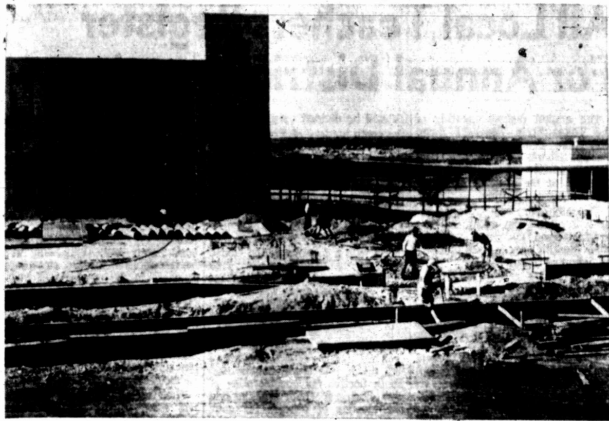
Major High School Addition
