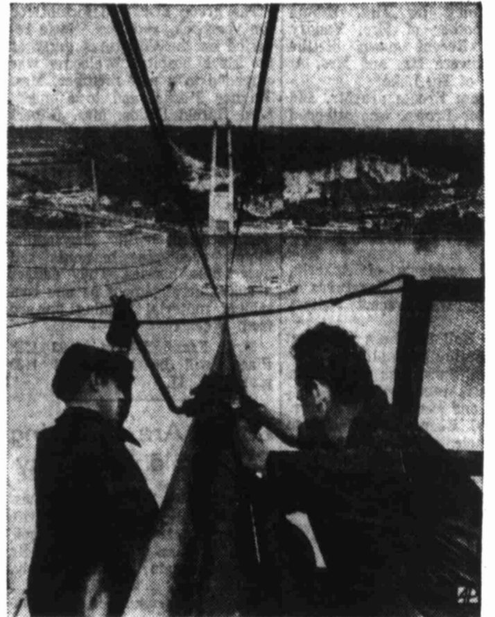
STEEL WORK — Workmen tighten cables for bridge under construction across Seine river at Pont Aude-mar, France. Bridge will be largest on European continent.
