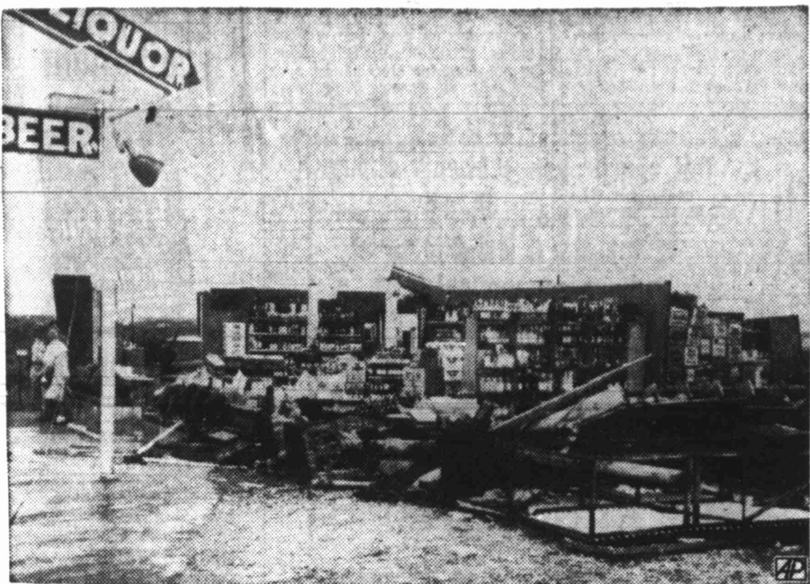
Only the Interior of the Pan American Liquor Store at Wichita Falls remained intact after a tornado struck, sweeping away the roof and walls of the concrete building. Damage was estimated at $50,000.
