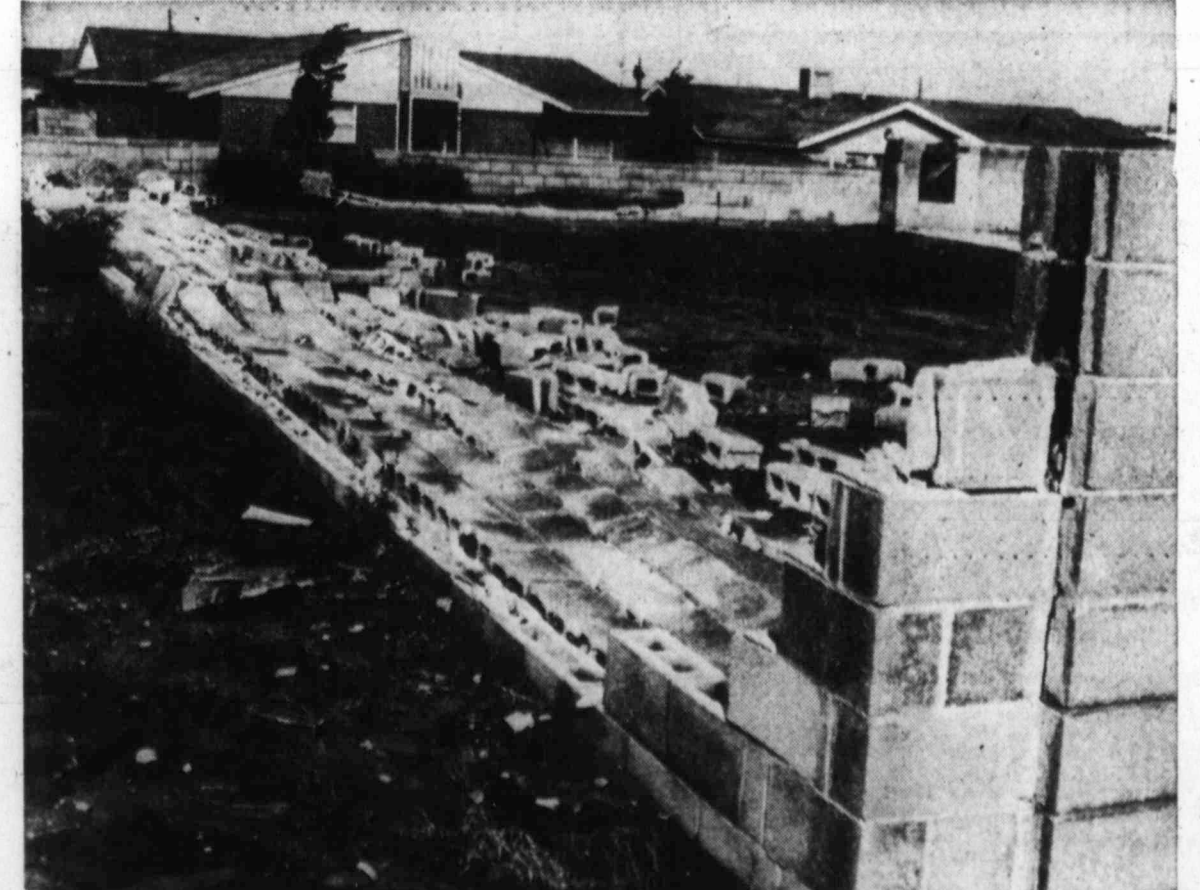
BLOCK FENCES TOPPLED BY STRONG WIND. Scene at rear of Rev. Ernest Stewart home, 710 Tulane
