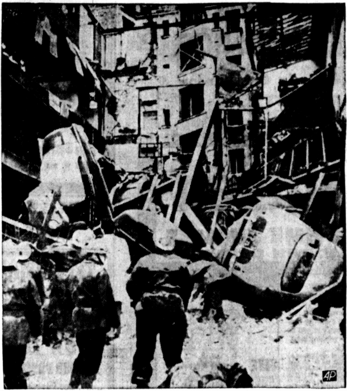
Explosion Shatters Paris Apartment House Firemen probe through the rubble following a gasoline storage tank explosion which shattered a seven story apartment building in Paris' crowded Montmartre section.
