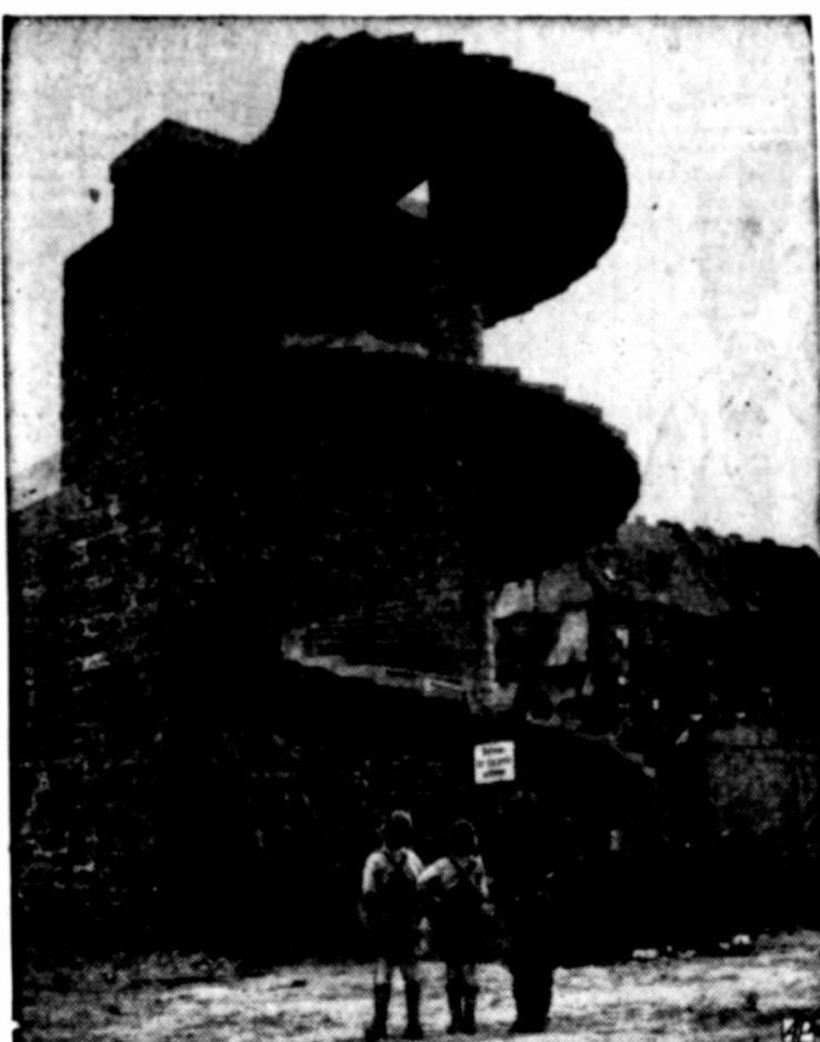
ABSTRACT TOUCH — Unfinished spiral stairway has an affinity to modern art and youngsters in Cologne, Germany. It was built as pedestrian approach to new Rhine bridge.
