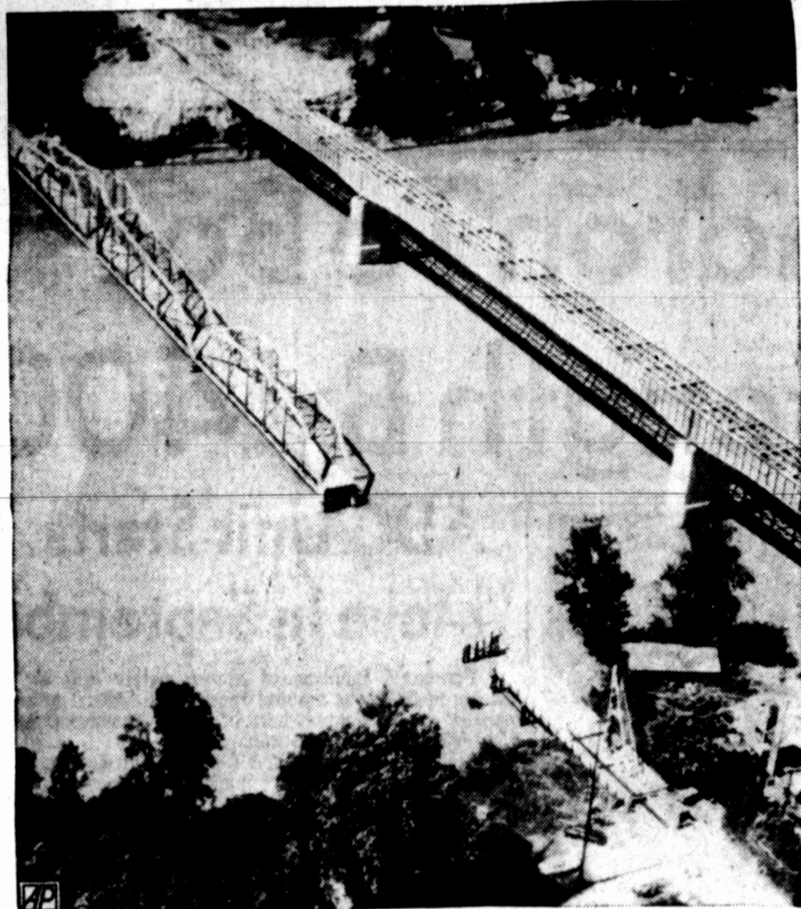
Bridge Washed Out
