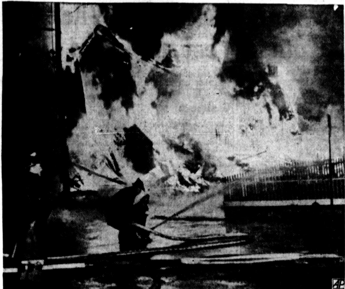
Walls Collapse During Fire
