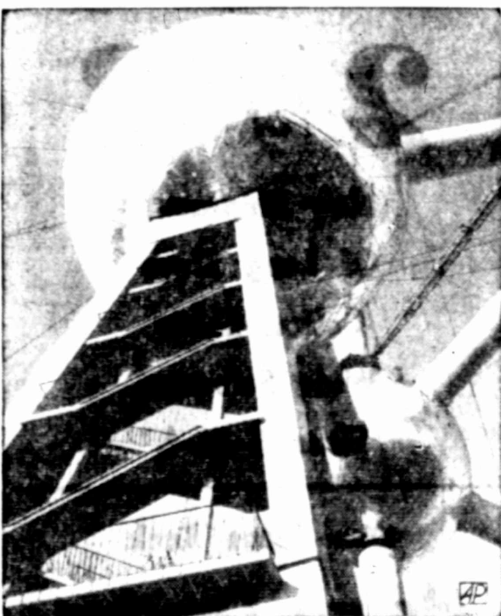
'ATOMS' SHAPE UP — Here's part of the nine-sphere Atomium nearing completion at the Brussels World Fair site. Each sphere, measuring 99 feet in diameter, houses exhibition halls. The connecting tubes house elevators and escalators.
