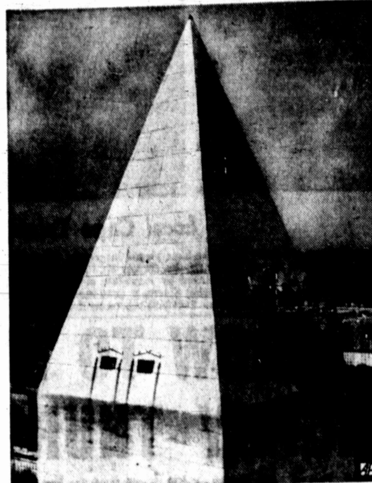
LOFTY WARNING — Workmen stand on temporary framework near peak of the Washington Monument to install a new lighting system which will warn off aircraft. View of peak, 555 feet 5 1/2 inches above the ground, was made from helicopter.
