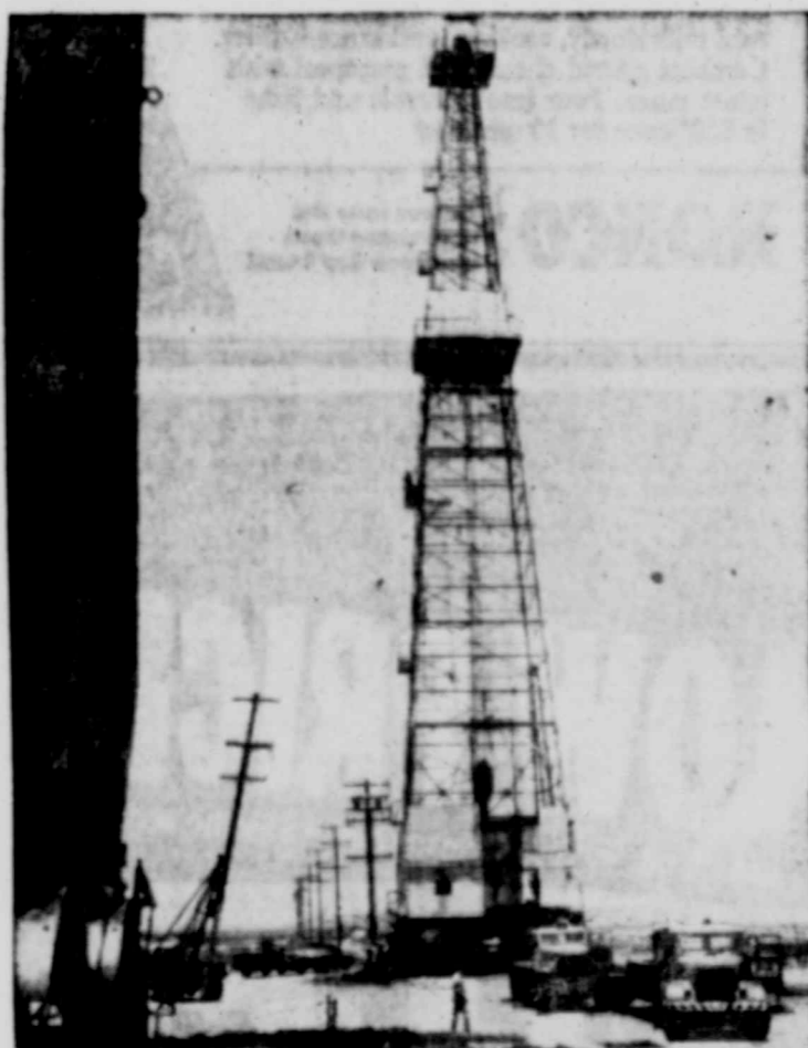
THE BIG TRANSFER — A sight not seen by many is a giant oil derrick on the move. Here's one being hauled by structural movers to new location at Huntington Beach, Calif.
