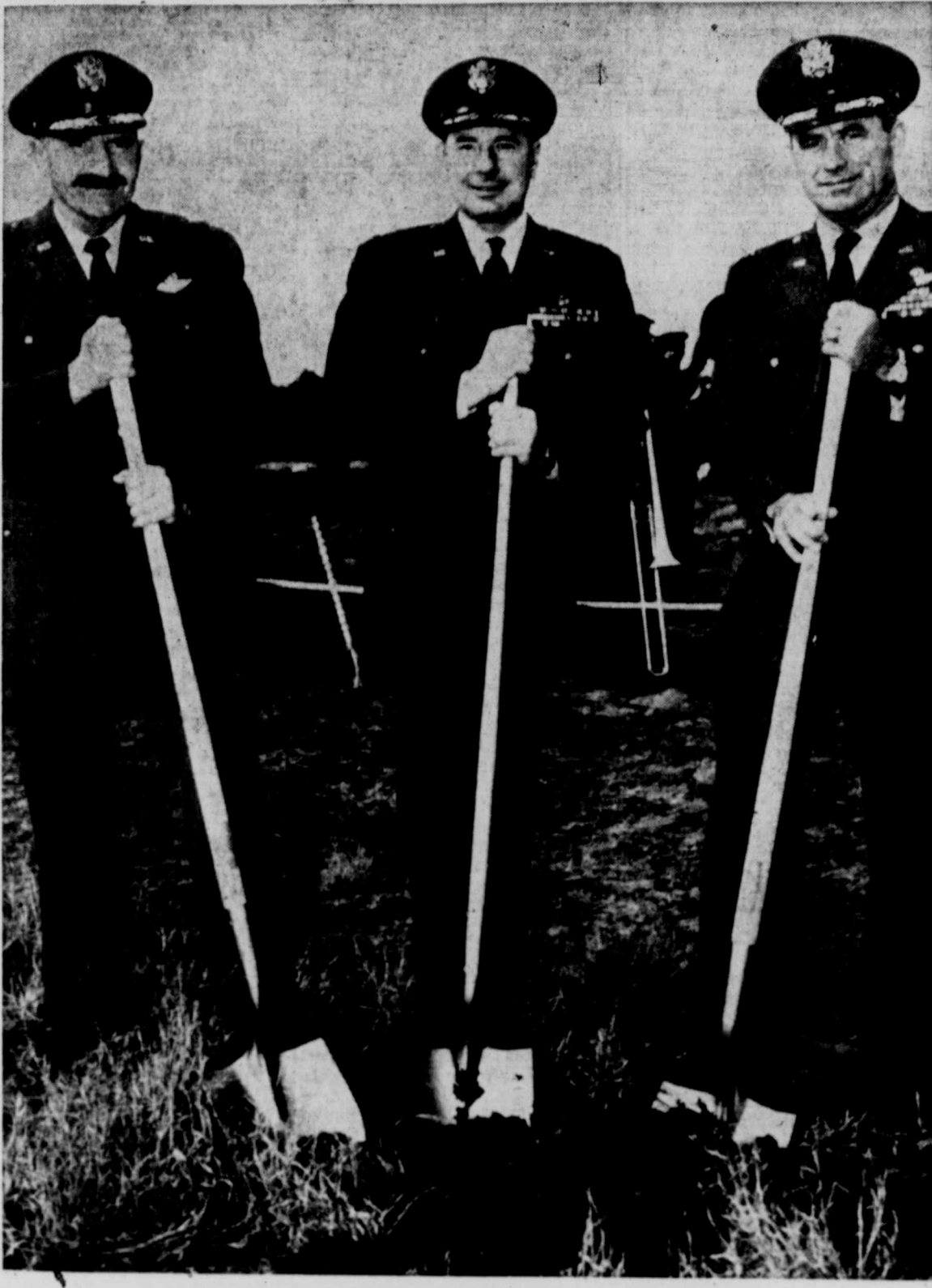
AIR FORCE LEADERS POISED TO START DIGGING Groundbreaking symbolizes start of big housing development
