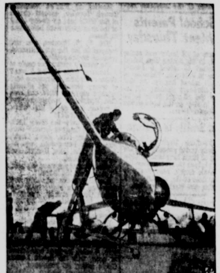
'NOSEY' TESTER — Snout on F104A jet is precision-instrumented boom to flight test the ultrasonic plane at Palmdale, Calif. Boom measures airspeed, pitch and yaw angles.
