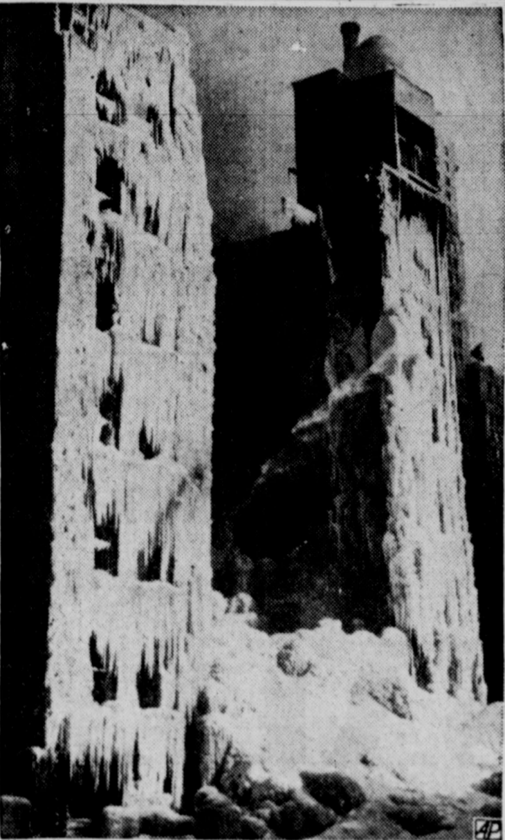
Cold Storage Building
