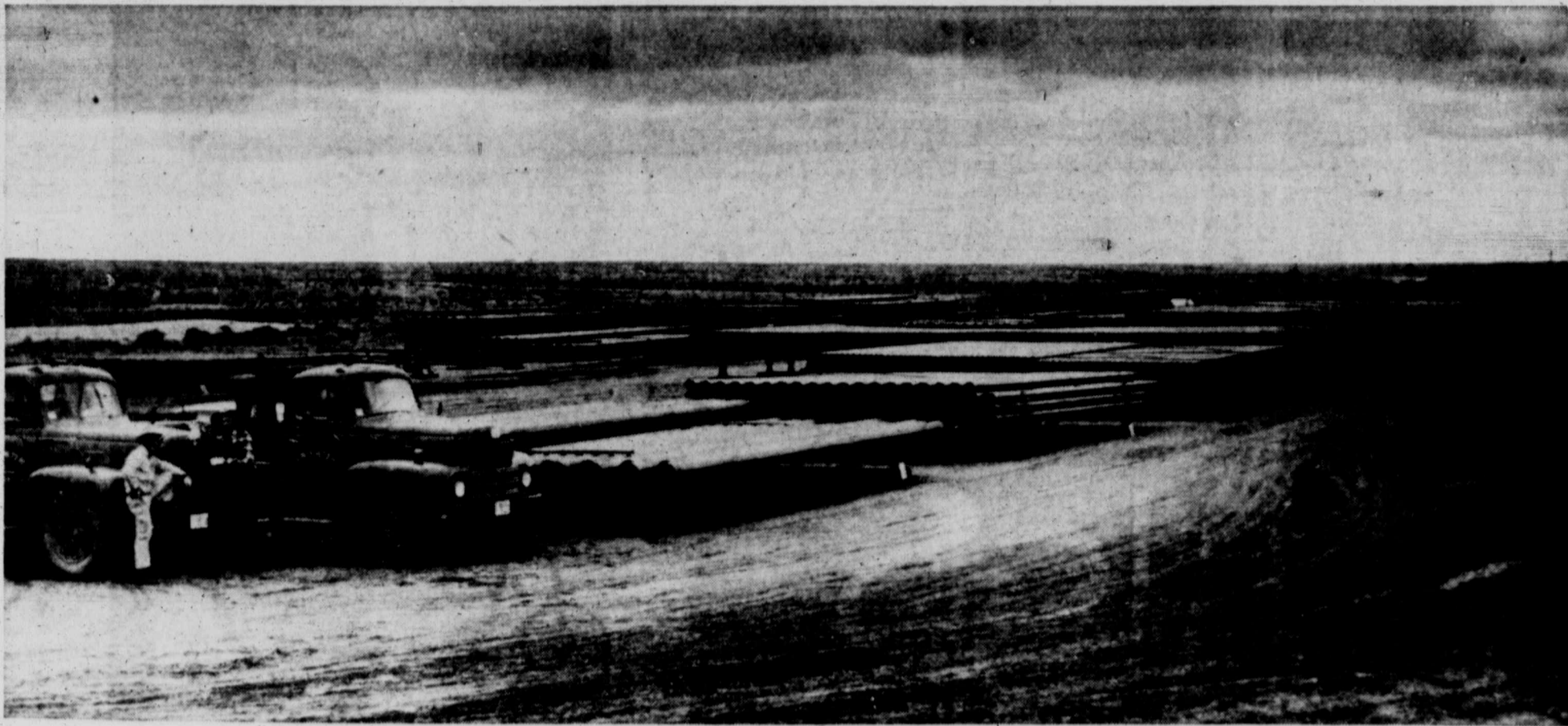
Acres Of Pipe At Storage Yard
