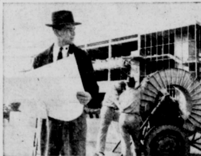
MORE NEW TELEPHONE BUILDINGS and equipment will be needed during next 20 years to meet what business forecasters say will be greatest period of growth ever. To assure financing, telephone company must maintain good earnings. Above, Construction Foreman Jim Doerr supervises as crew gets set to reel out new underground telephone cable.
