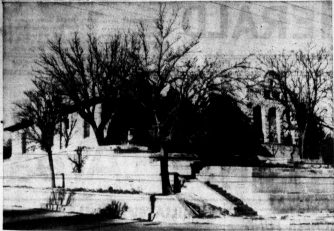
Landmark To Serve New Purpose
