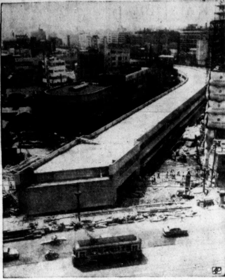
Road Above, Building Below
