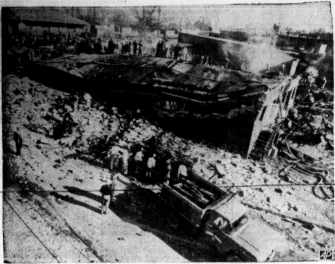
Blast Levels Buildings
