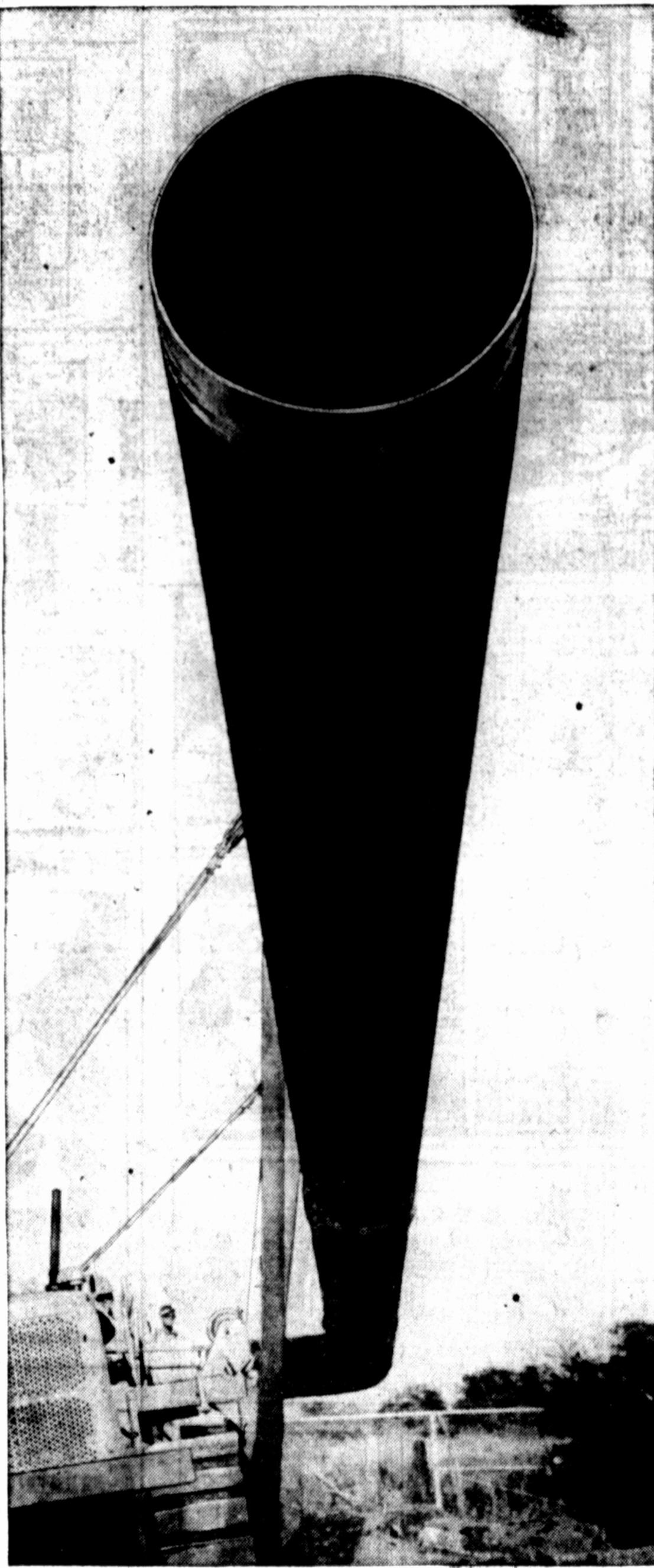
Giant oil pipeline under construction. Photo courtesy Cities Service Company.
