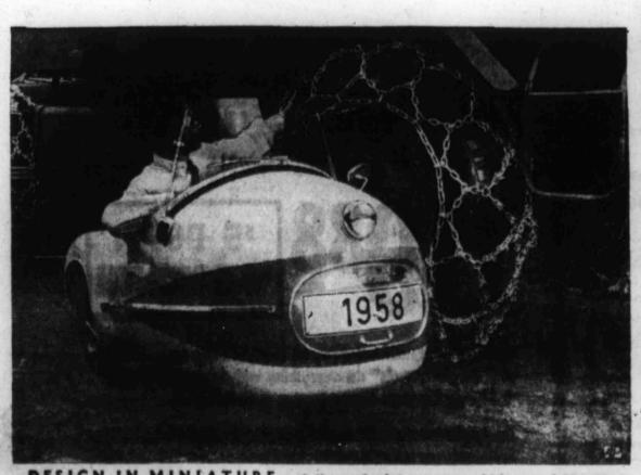
DESIGN IN MINIATURE — A three-wheeled one-man vehicle named Mopetta is dwarfed by huge wheel of another vehicle at Frankfurt exhibition. The German-manufactured car has 2½ horsepower air-cooled engine, can cruise at 27 miles per hour and sells for \$250.
