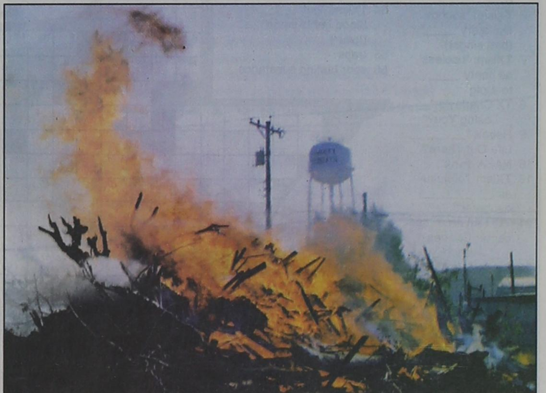
AFTER THE CITY, with the owners permission, demolished this house in the southeast part of town on Aug. 13, it was destroyed with a controlled burn the next day.
