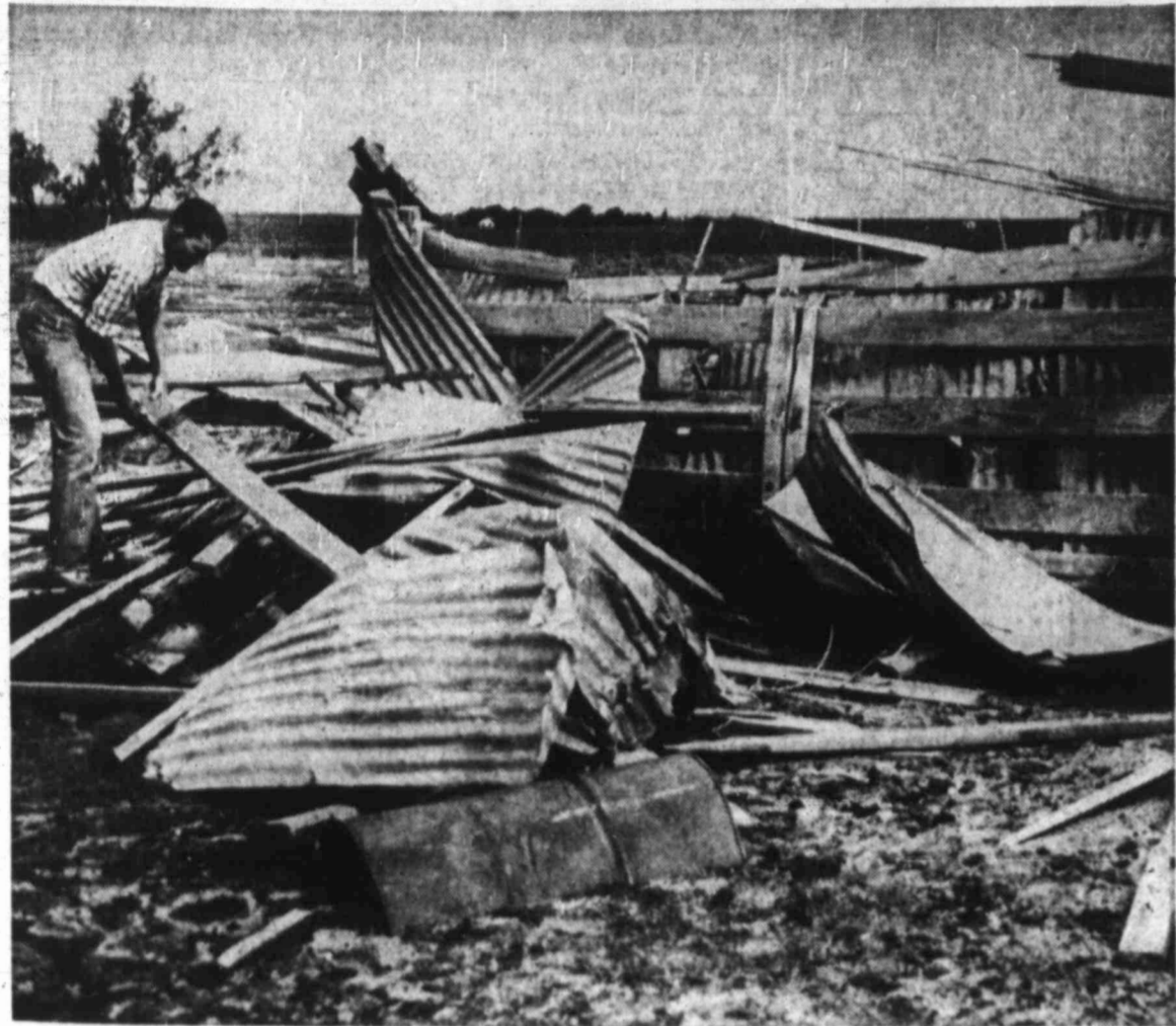
Wind Damage At Elbow
