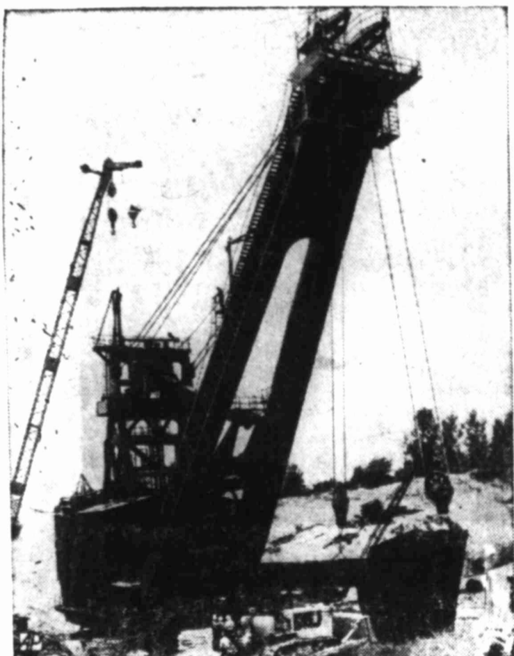
'BIG BITER' — Workmen ready a huge coal stripping shovel at Freeburg, Ill. The giant jaws can strip 150 tons of dirt or rock with one cut to lay bare a vein of surface coal.
