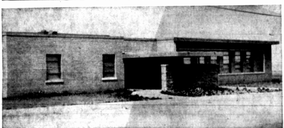
MUSIC BUILDING AT HCJC Structure incorporates all modern features.
