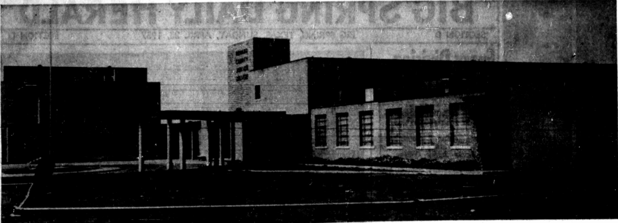
ADMINISTRATION BUILDING, FLANKED BY AUDITORIUM, LIBRARY Wing at right was provided out of $600,000 bond issue last year.
