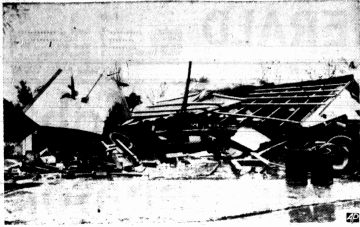
Tornado Levels Garage
