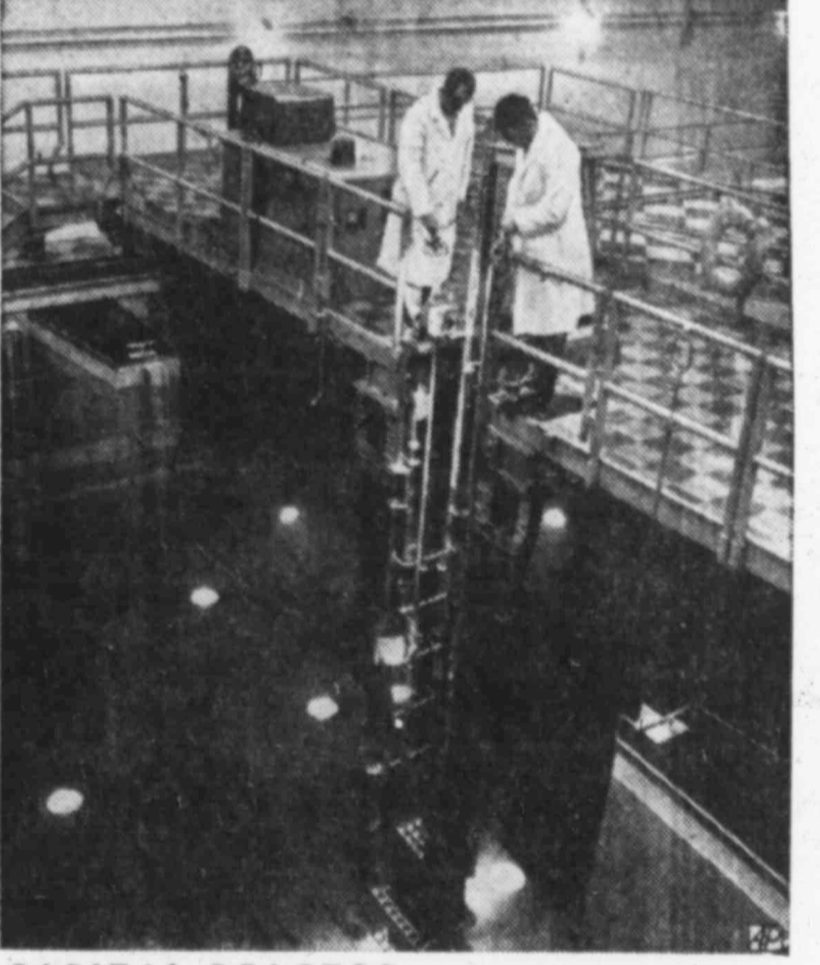
CAPITAL REACTOR — Fuel elements are loaded into core of new nuclear reactor in pool at Naval Research Laboratory in Washington. It provides neutrons needed for research.
