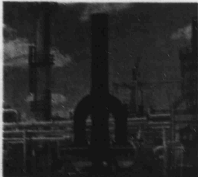
To meet the challenge of new higher-compression engines, Cosden built the world's first fully-integrated Raxformer. This $2½-million plant utilizes a completely new process to yield higher-octane gasoline, more than matching the requirements of today's newest engines.
