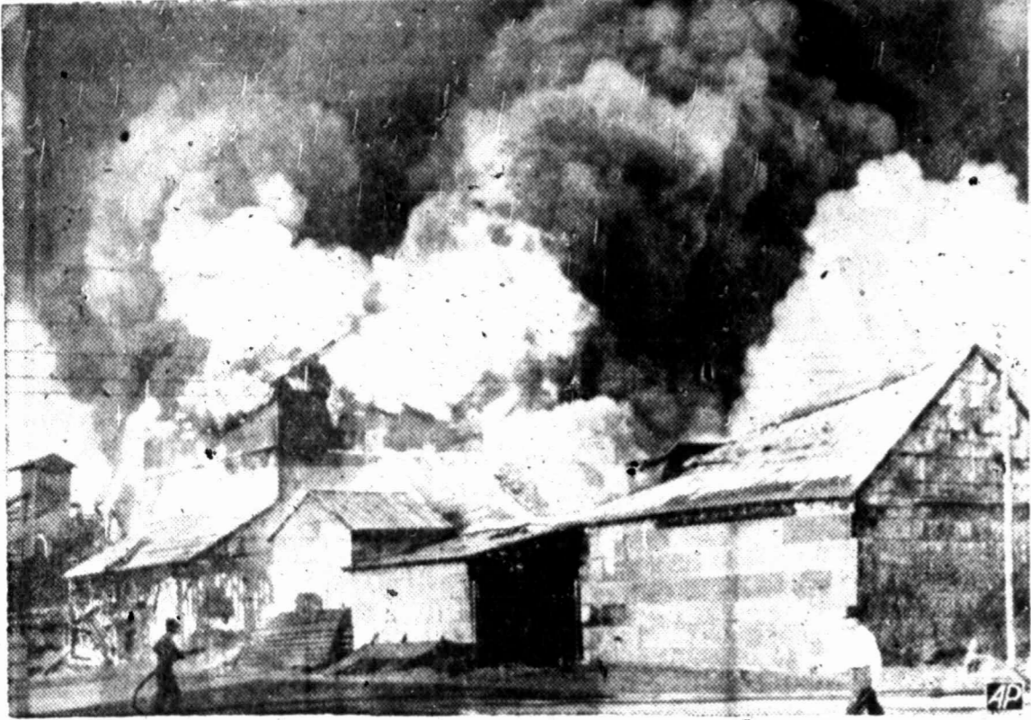
Grain Elevator Fire
