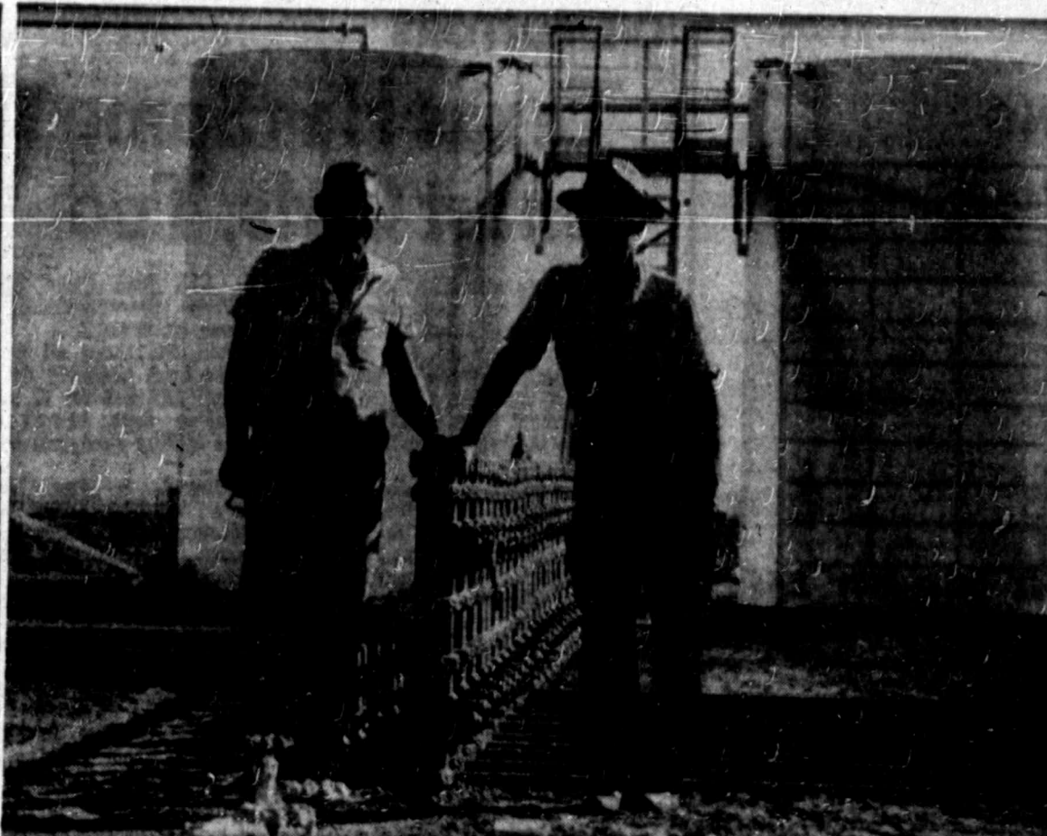
Production Men At Manifold
