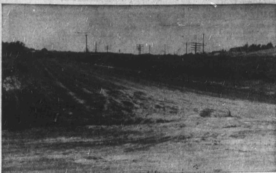
First Street Canal
