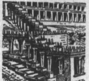
A portion of the Grand Stairway (reconstructed).
