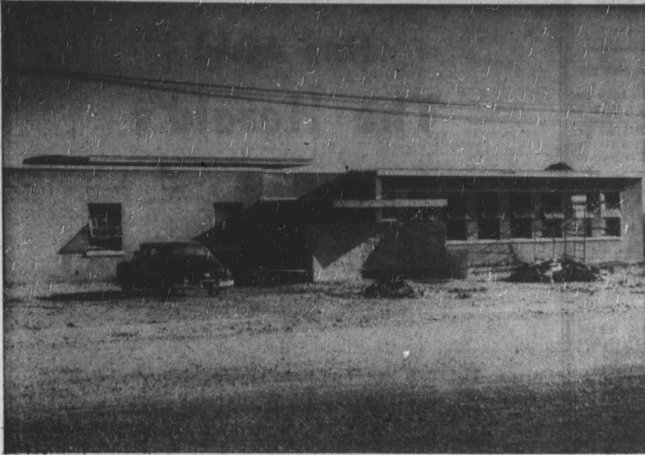
Pictured above is the new Music Building that will be completed September 1.
