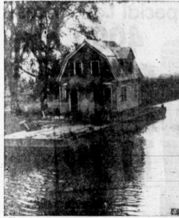
CANAL STREET —A seven-room house purchased by Henry Van Hervele is moved from near Geneseo, Ill., to his farm at Green River via Hennepin Canal barge towed by truck.
