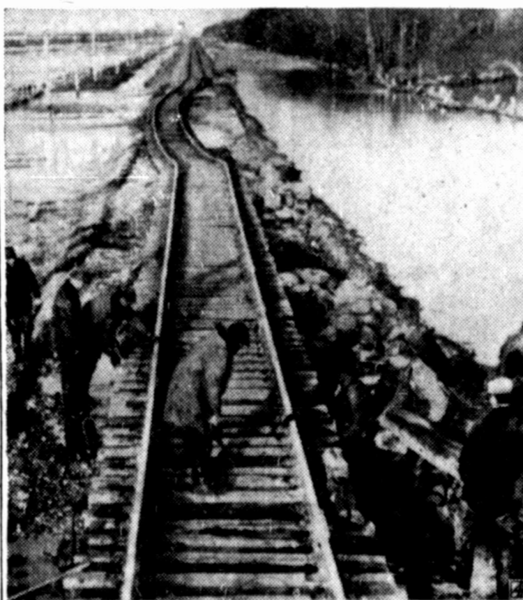
Track Washed Out
