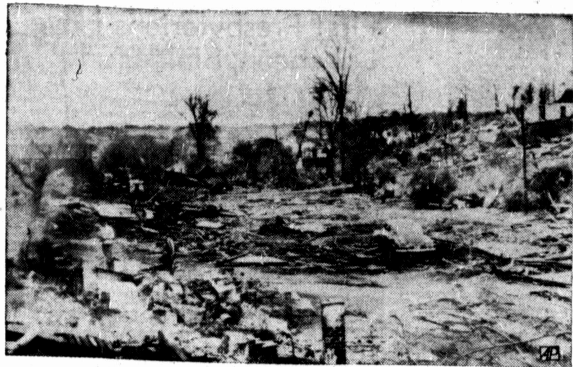
Entire Neighborhood Blown Away
