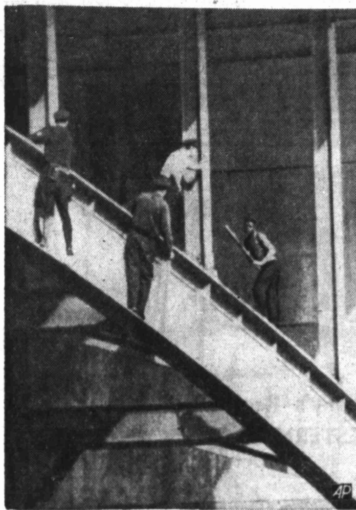
At Bay On Bridge
